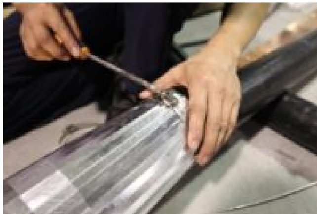
Installation of HLVJ-4-A-M-D
